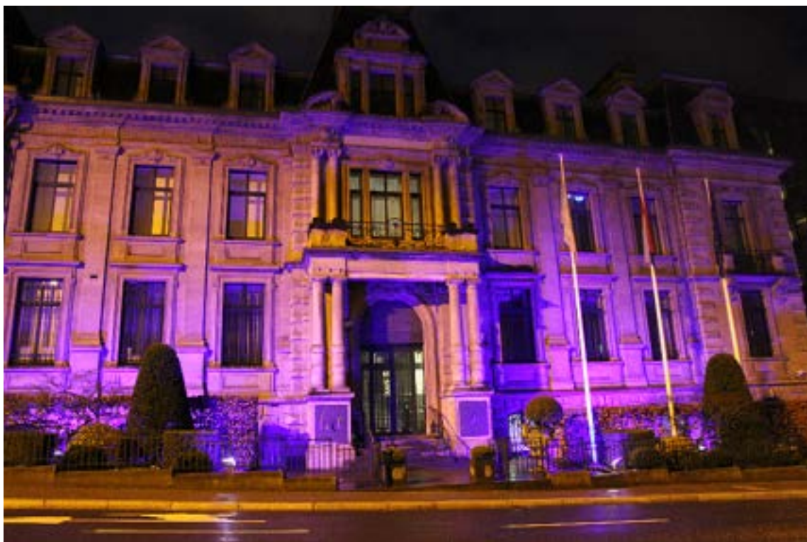
Illumination of the facade of the historic building in blue.
